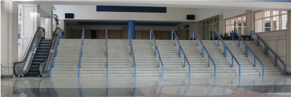
Left #32 and Right #34 Staircase — Total: 15 risers each 50'-6" w x 6 1/4" h
